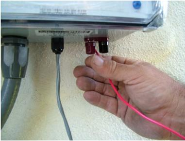
1.) Insert the pre-stripped end of the signal cable into one of the two binding posts located on the bottom of the control box. It does not matter if you hook it up to the red or the black binding post. The receptacle post can be unscrewed by turning it counter-clockwise. This will expose a small hole in the post. Tighten the receptacle post as much as possible with the signal cable completely threaded through the hole.
