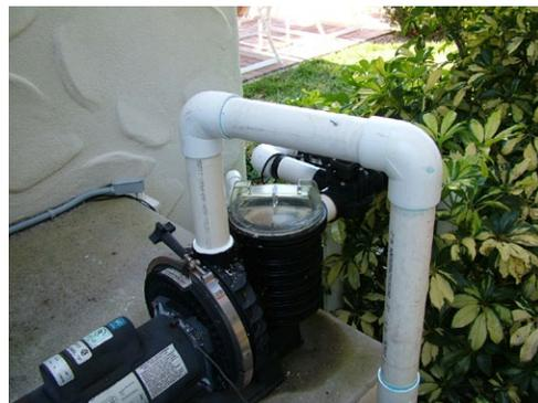
3.) Locate a space to mount the black flow-cell chamber. **Always install on the return line.** If possible, install the chamber after the filter, but it is not required if there is not enough space. If necessary, you can re-pipe an entire section to allow proper room for the electrode chamber or **ScaleBlaster** coil.
