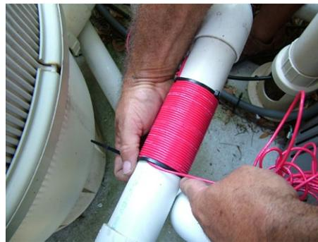
5.) Route the loose end of the signal cable back to the power unit. Trim the cable to length. There may be several feet of unused wire. This extra wire was included in case the control box was mounted several feet away from the return line.
