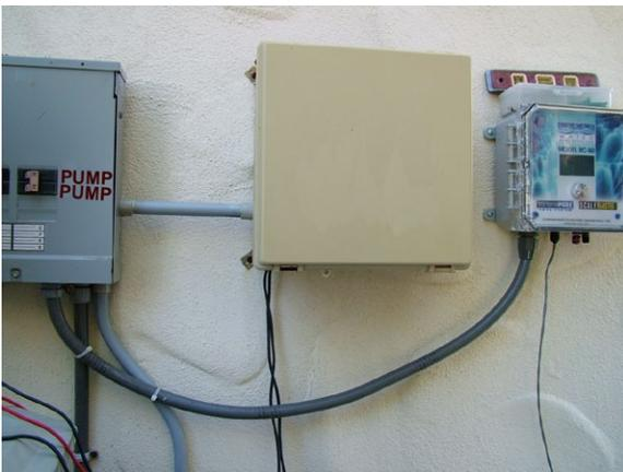
You should use a flexible conduit from connection to connection on the power cord to meet codes. The size of the connector already on the control box is 1/2". There is no need to cover up the electrode wire with conduit.
