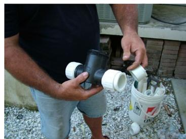
2.) If the pipe size where the flow-cell chamber is being installed is 1 ½”, glue the two reducer bushings (2” x 1 ½”) into the male adapters. This step is not necessary if installing on two-inch pipe.
